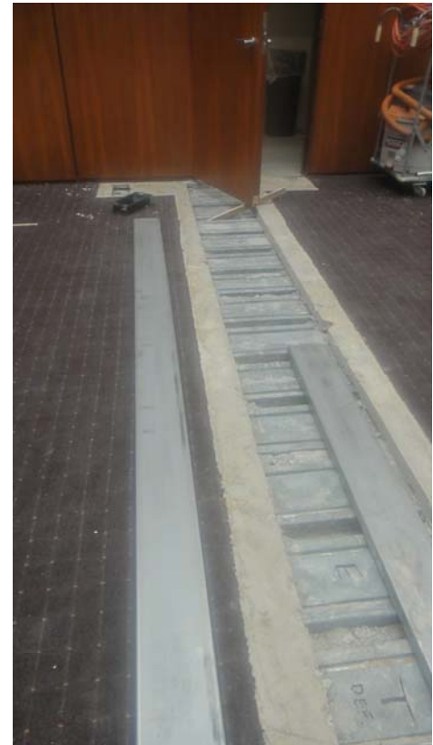
Exposed Trench-Duct prior to lid and carpet covers
