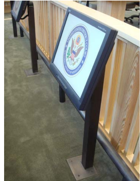
Mount for jury box display where Jury rail mounting is not an option
