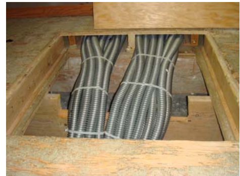
AudioVisual FMC used where EMT would have been more appropriate
