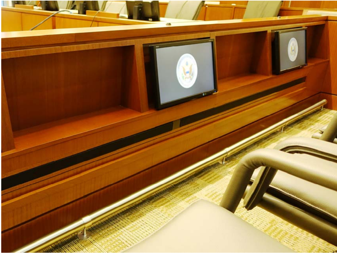
A Contemporary Jury Box where the Casework is designed for the Displays. Note Built-in Speaker Strips below Displays
