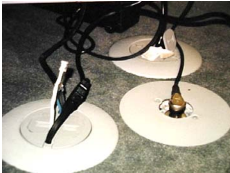
Typical round Poke-Through Device. Note that the trim is not flush to the floor and that connectors must stick up where they are susceptible to damage
