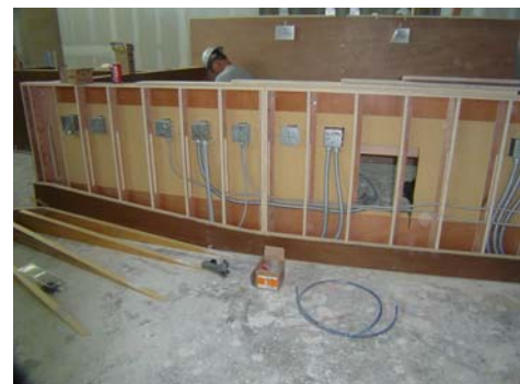
Partial conduit rough-in for a jury box
