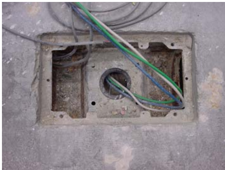
Typical Trench-Duct activation point
