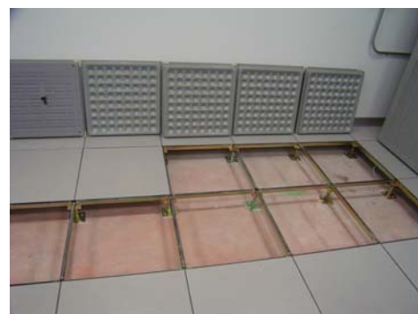
Access Floor being installed in an Equipment Room
